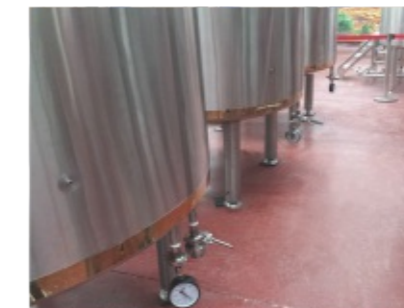
试压 Pressure Testing
